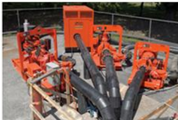
Bypass Temporary bypass pumping
